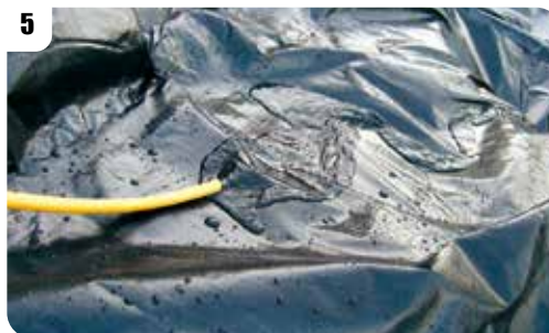
5 Fill pond with water. We filled ours straight from the mains via a hosepipe.
