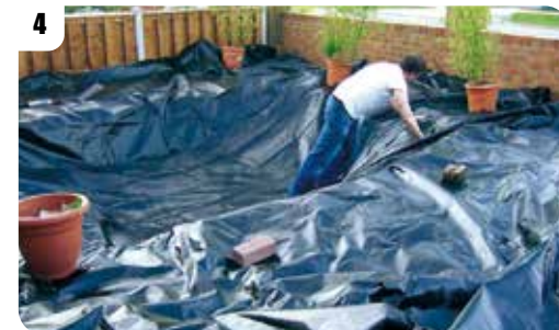
4 Once the liner has been unfolded it's time to smooth it into the shelves and corners as best you can (barefoot is best).
