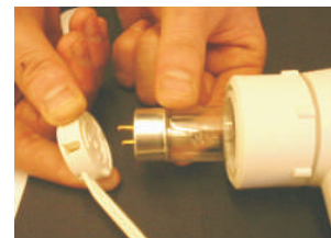
5). Disconnect lamp holders and remove lamp
