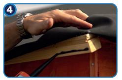
**Apply a bead of edge sealant** and press the membrane onto it. Once dried this will hold the membrane securely.
