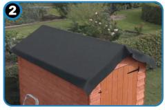
**Apply the rubber membrane** by laying it in position on the roof for 20 – 60 minutes. Fold the membrane back to the centre of the roof ready for adhesive.
