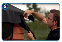
**Remove any excess membrane** using scissors. If an edge trim is used, install this first then use the underside of the trim as a guide to cut the membrane.
