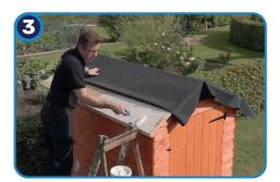
**Apply the adhesive** to the entire roof working 'in stages'. Roll the membrane gradually onto the adhesive whilst wet.
