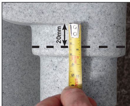
10. On the inlet, measure 20mm down from the shoulder of the inlet section.
