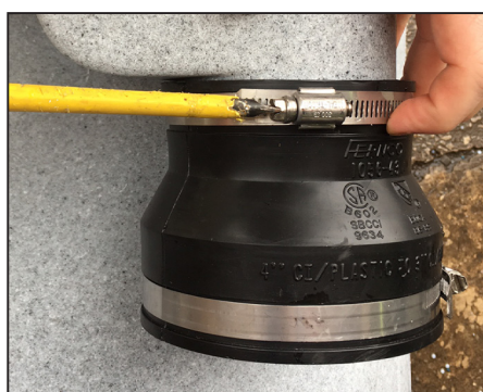
15. Tighten up the jubilee clip using a flat head screwdriver.
