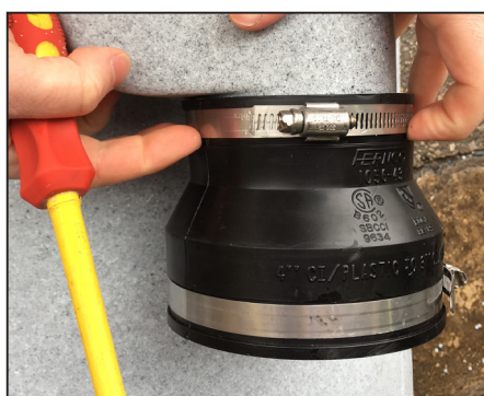
13. Fit the 4" to 3" EazyConnector onto the inlet you have just cut.
