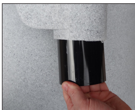
12. Inside the inlet, there is a black pipe which you should pull out of the inlet.
