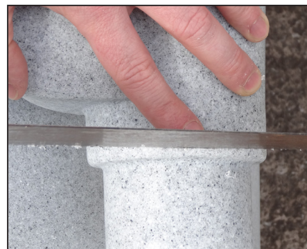
11. Using a hacksaw, cut across the inlet at the measurement shown.
