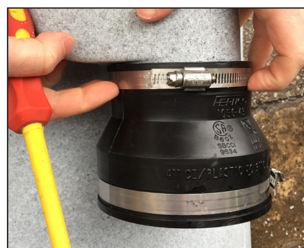
14. You will need to loosen the jubilee clip on the 3" side and slide this up to ensure a tight fit.
