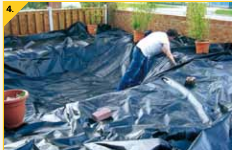
4. Once the liner has been unfolded it's time to smooth it into the shelves and corners as best you can (barefoot is best).
