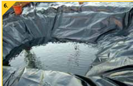
6. Weigh liner edges down then smooth away folds as water starts to fill the pond.
